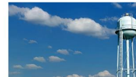
Water and Wastewater Systems
